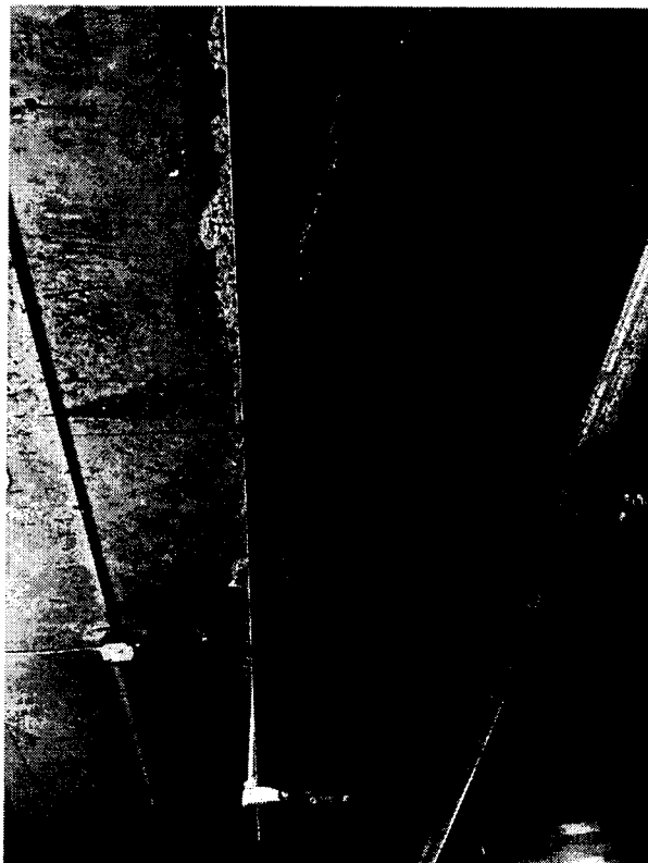
Photo 2: W18 Girder Exhibiting Bottom Flange Rust at Midspan
