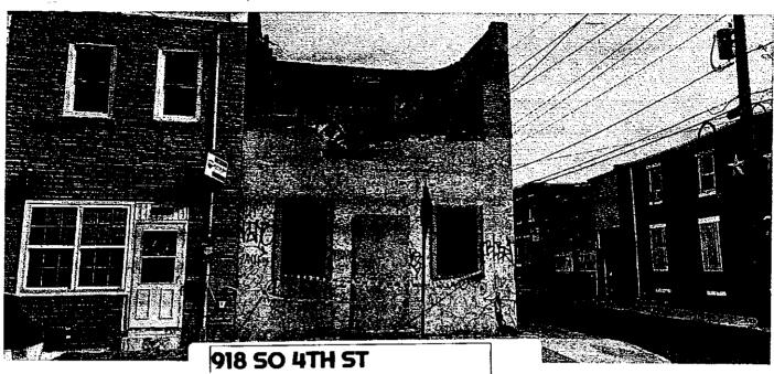
918 SO 4TH ST TOTAL ROOF COLLAPSE SEVERE WALL FRACTURES
